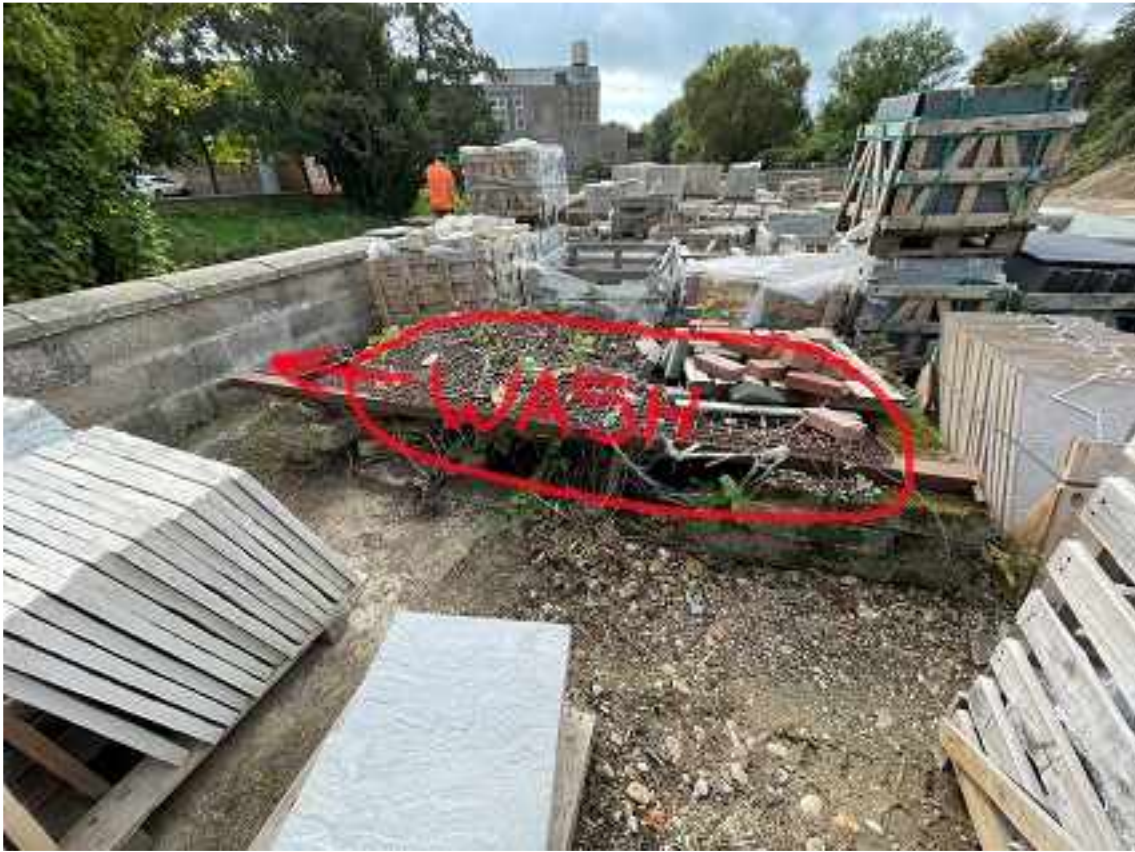
REDUNDANT WASH PIT
